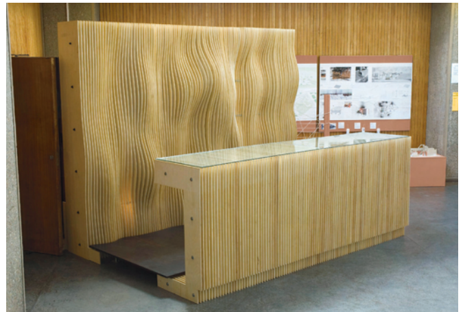
'Centenary Bar' at Sheffield University's School of Architecture, CNC machined Grade S/BB Birch Plywood with WISA-Hexagrip floor.
